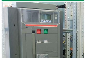
Sends trip signal to breaker trip coil (undervoltage or shunt trip) to interrupt power. Ability to trip upstream breaker if local breaker fails.
